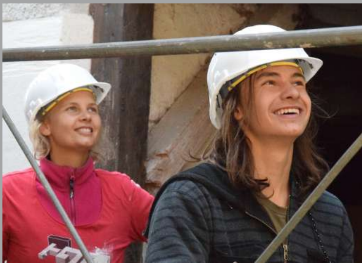
Workcamp „Animal Sanctuary Renovation Works“ in Kleinlützel SO (Luglio 2019)
